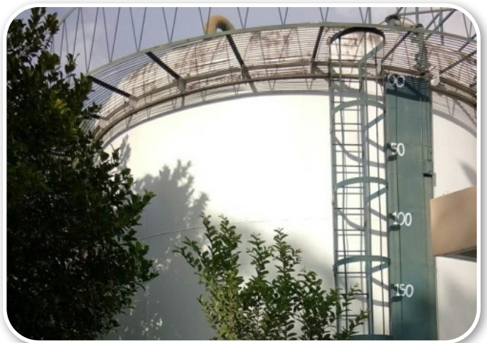
EMILY Ground Reservoir and Booster Station
